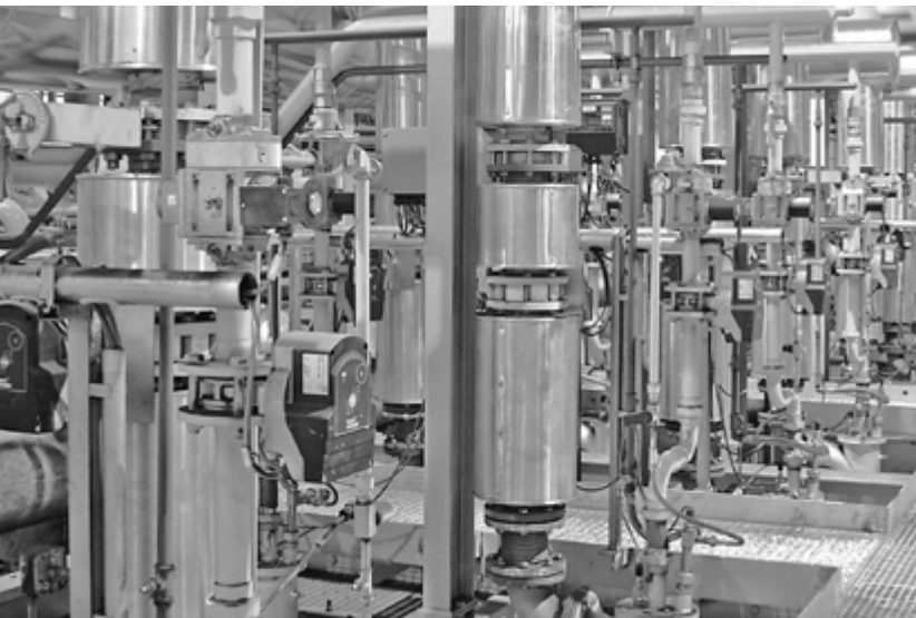
Walking beam furnace with overhead firing
